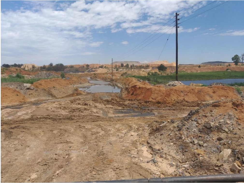
Figure 8: Water attenuation on access road across watercourse.
