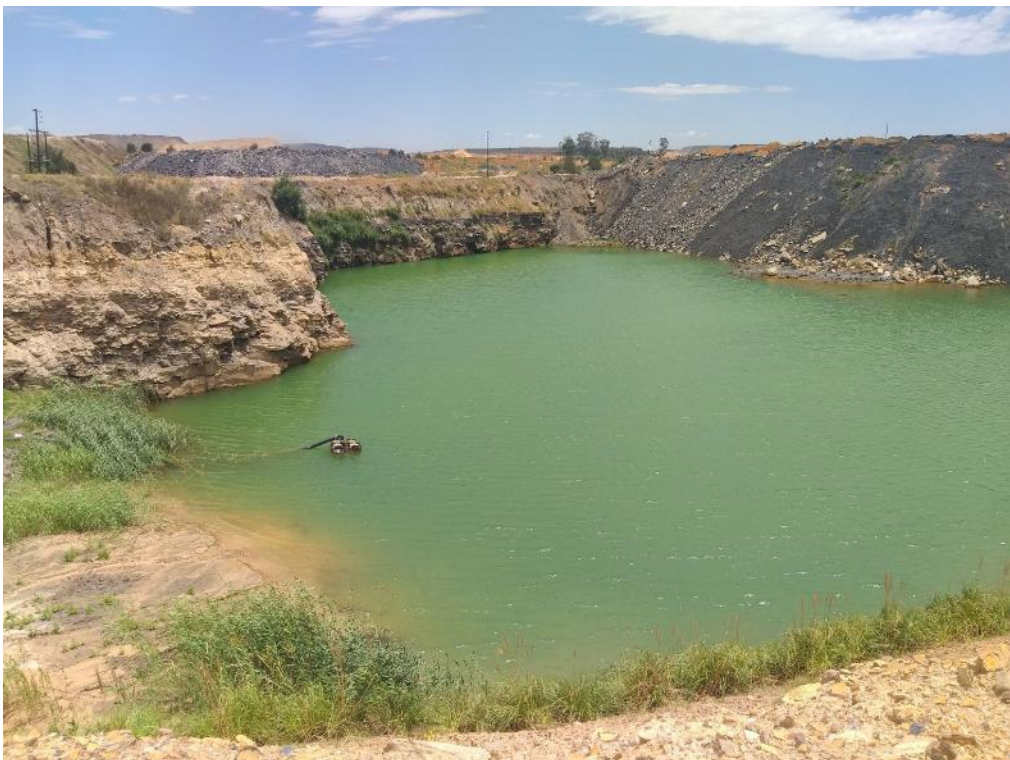
Figure 7: Western Opencast Pit void used for containment of runoff water.
