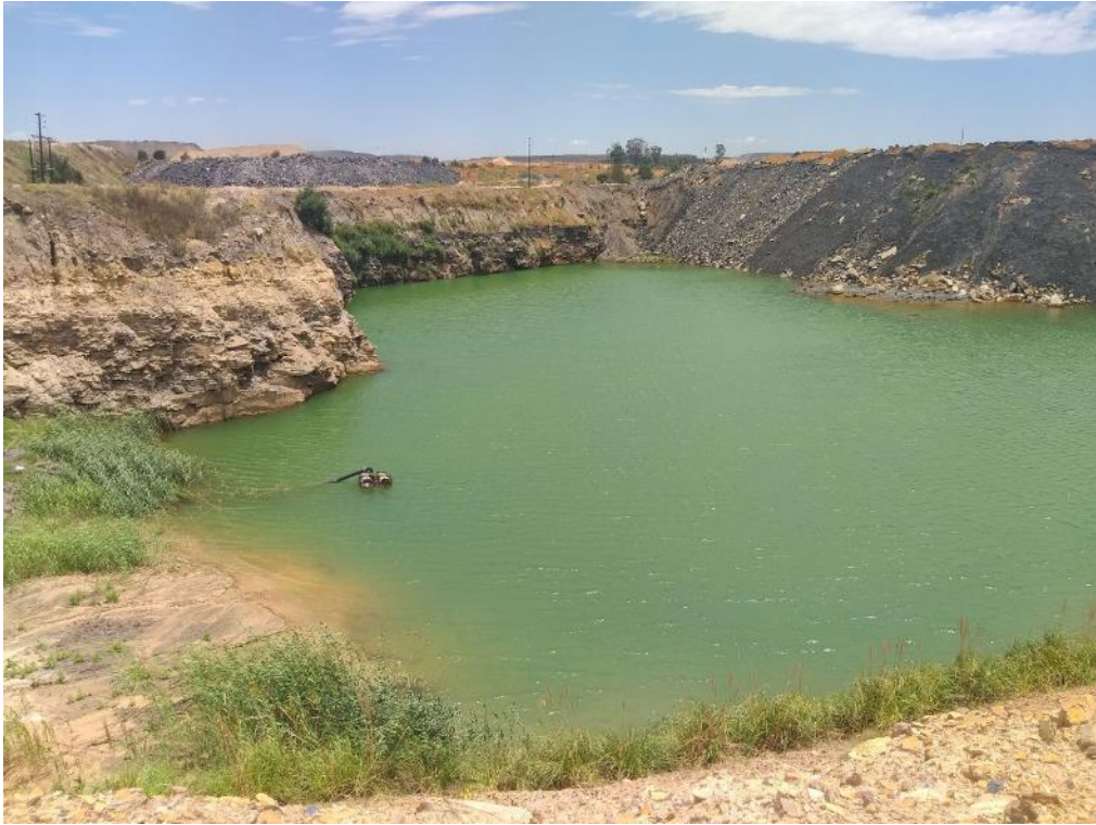
Figure 10: Western Opencast Pit used for containment of runoff water.
