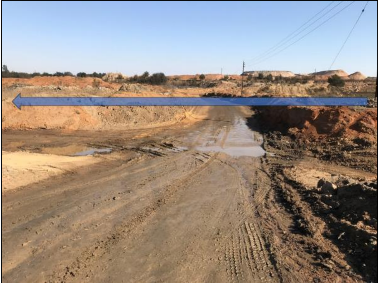
Figure 21: Example of a wetland crossing (blue arrow indicating position and direction of flow)
