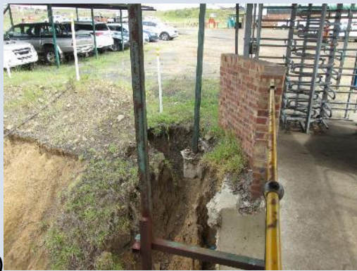
Figure 3: Erosion at the storm water drain to the east of the offices (a), north of the shaft (b) and on the subsoil stockpile (c).
