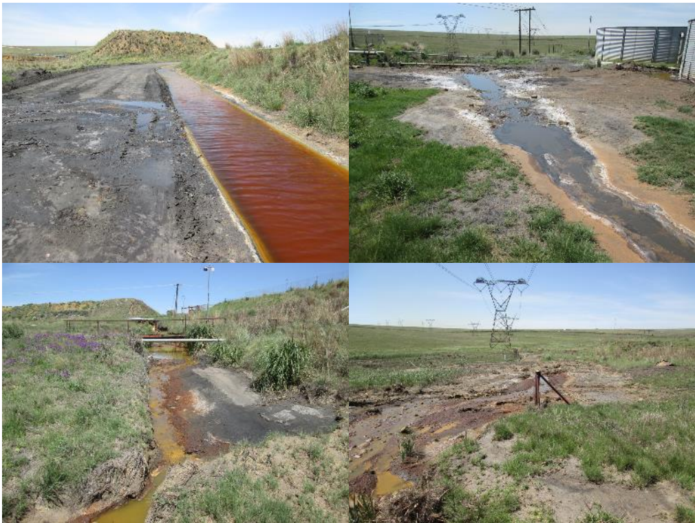
Figure 12: Concrete trench around the co-disposal overflowing towards the watercourse to the south-east of the mining area.
