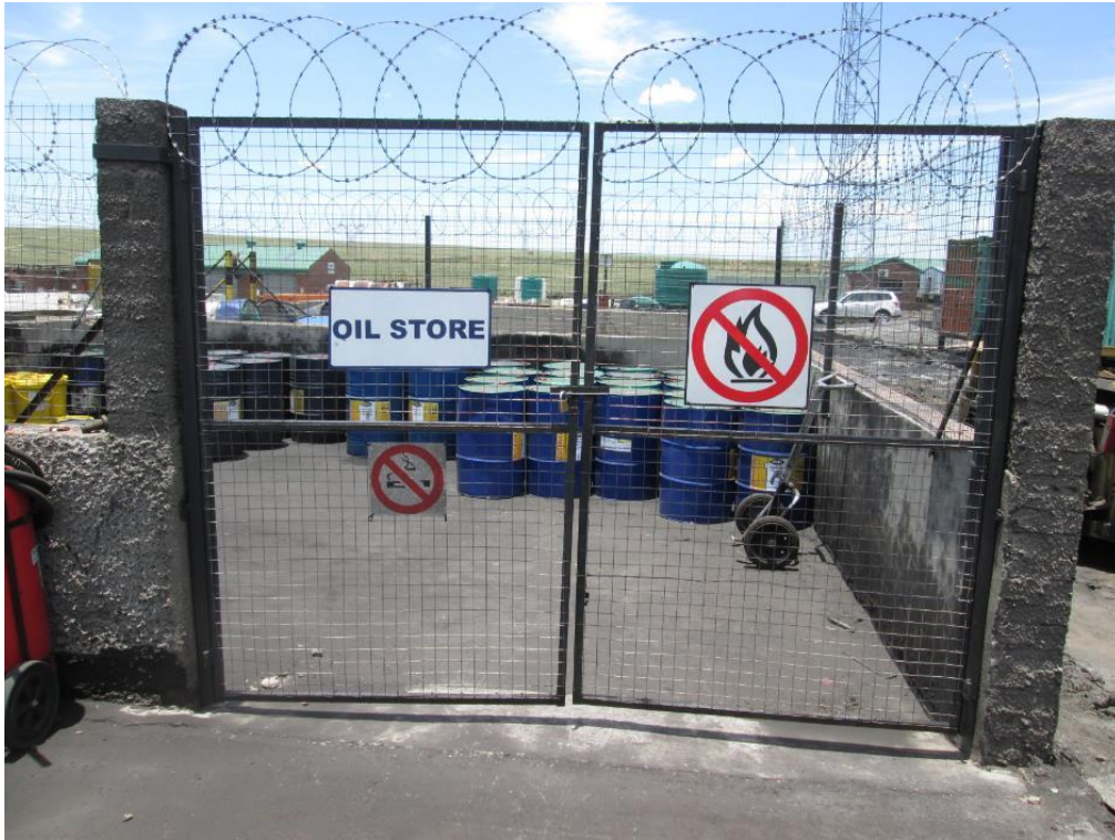
Figure 15: Designated hazardous storage area that was lined, access controlled and signposted.
