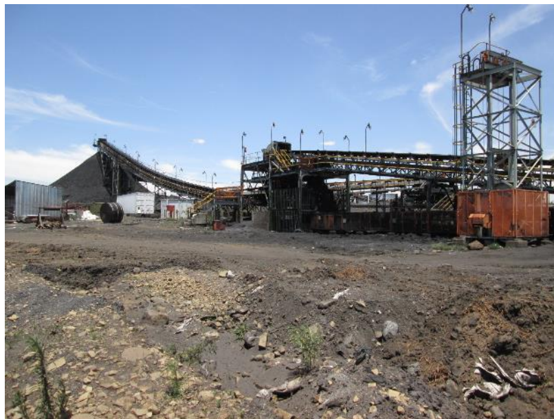
Figure 7: Spills from the ROM conveyor.
