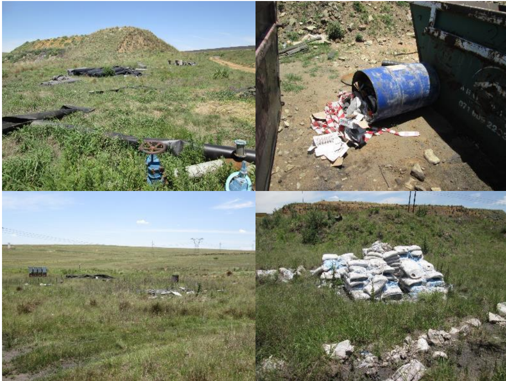
Figure 13: Housekeeping concerns at Mooiplaats Colliery.
