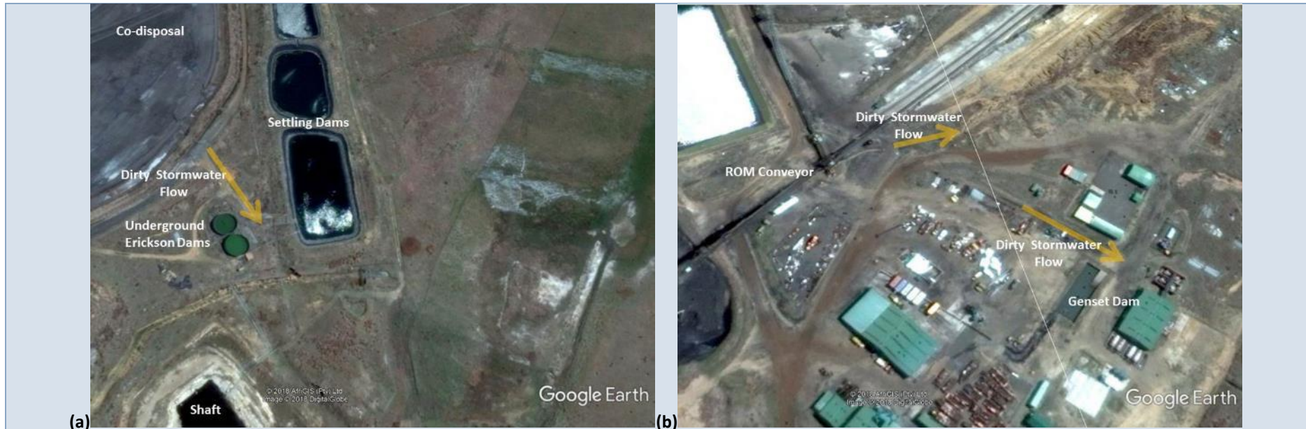
Figure 4: Uncontained dirty storm water from the co-disposal facility (a), ROM conveyor, workshops and laydown area (b).
