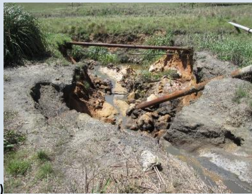
Figure 3: Erosion at the storm water drain to the east of the offices (a), north of the shaft (b) and on the subsoil stockpile (c).
