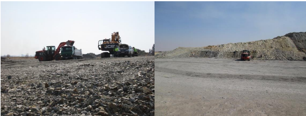
Figure 9: Removal of waste rock dump.
