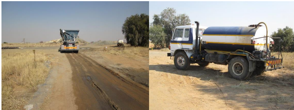
Figure 7: Dust suppression on access roads.
