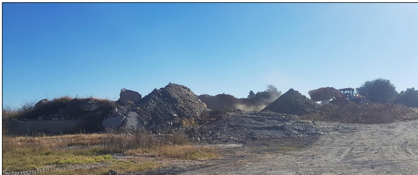
FIGURE 1-3: BACKFILLING OF THE OLD SHAFT USING WASTE ROCK
