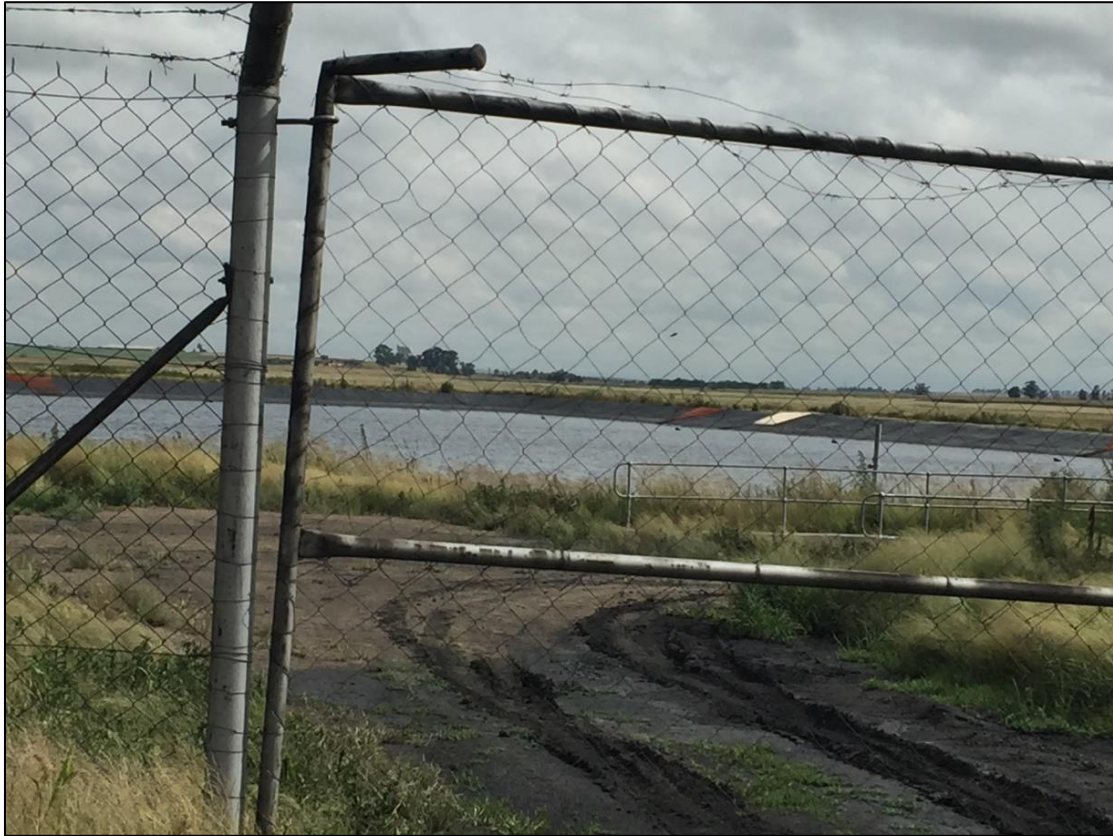
Figure 6-5: Manungu Pollution Control Dam
