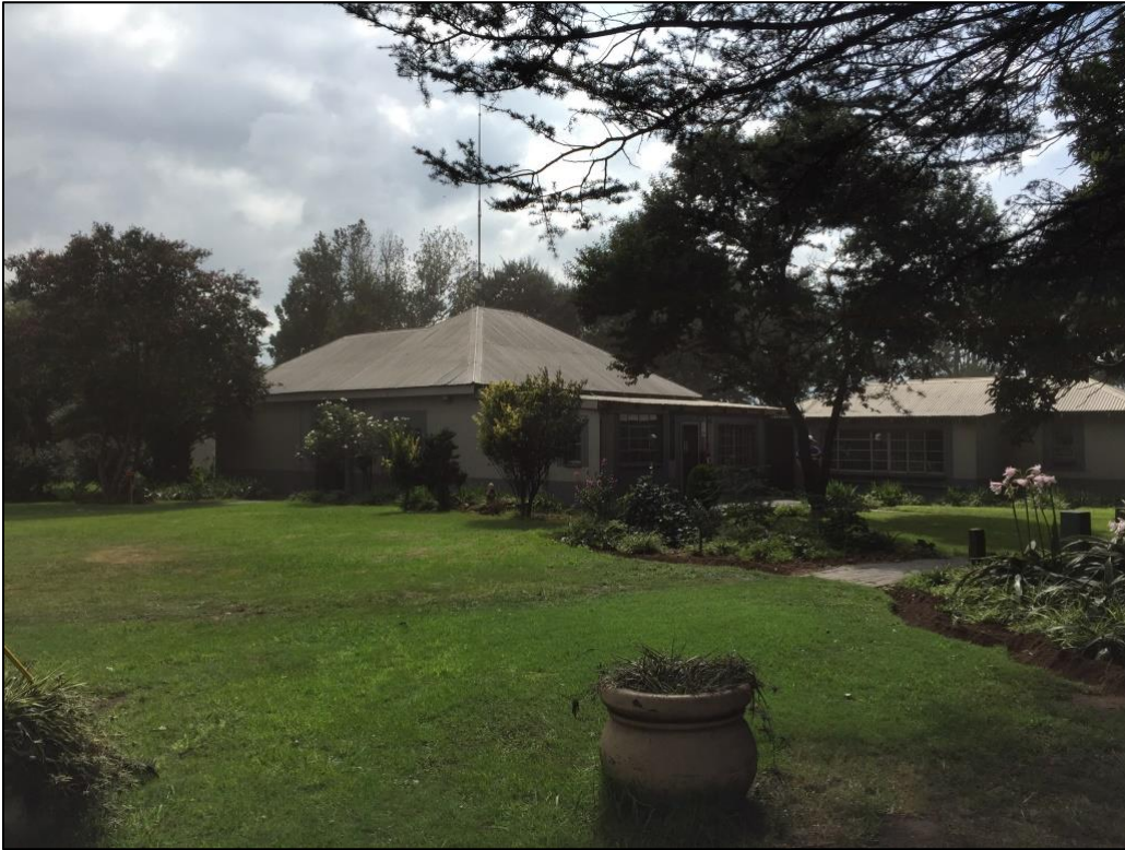
Figure 6-1: Main Office Building
