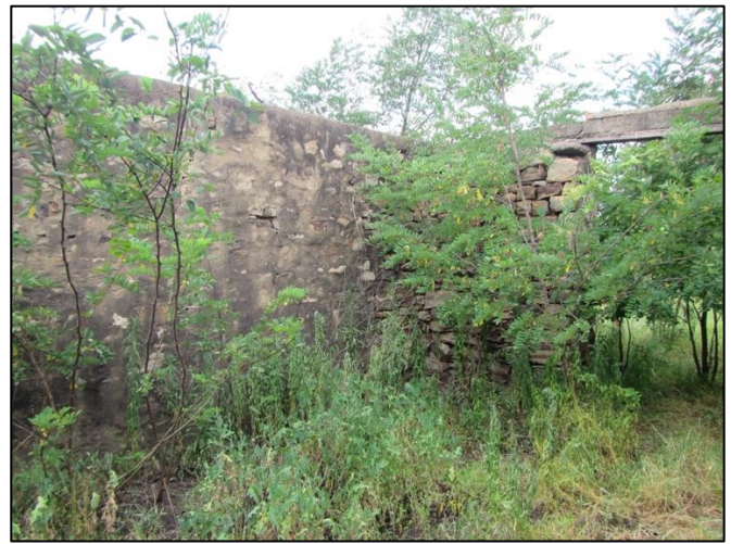
Figure 32 – MN009 within the stone building
