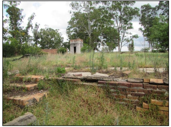
Figure 30 – MN009 general view
