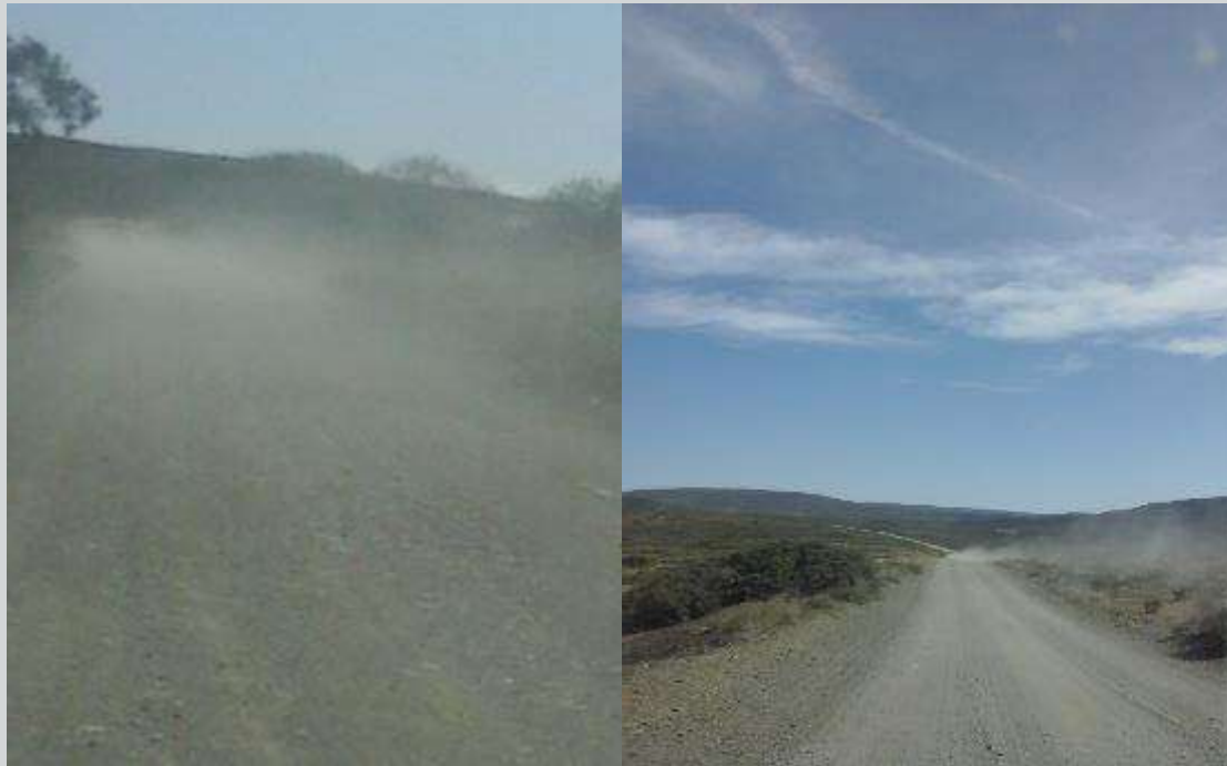
Figure 3: Dust emissions from vehicle movement on access roads with no dust suppression measures in place.
