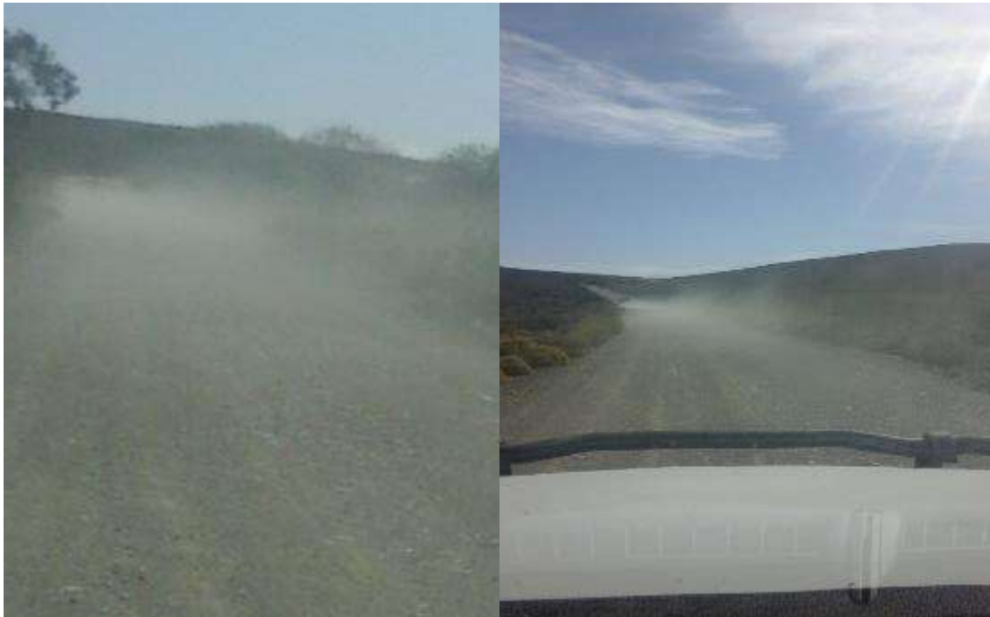
Figure 4: Dust emissions on access road and no dust suppression measures are being implemented.
