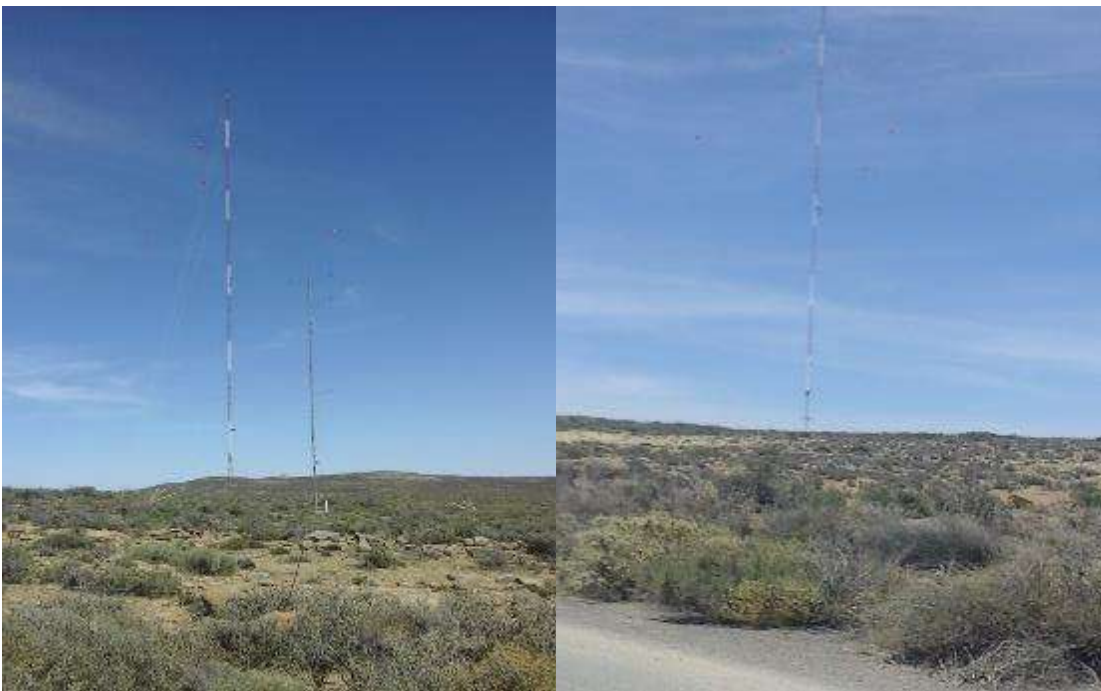
Figure 9: Signal and weather antennas observed within construction footprint during the audit.
