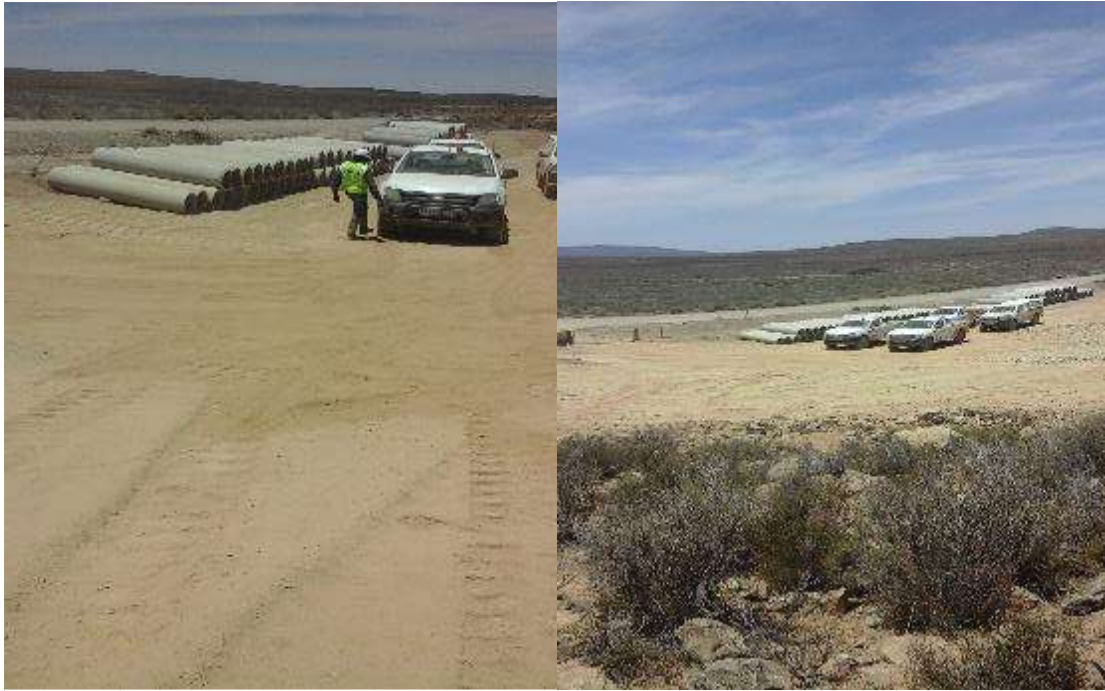
Figure 12: Pipe laydown observed during the audit.
