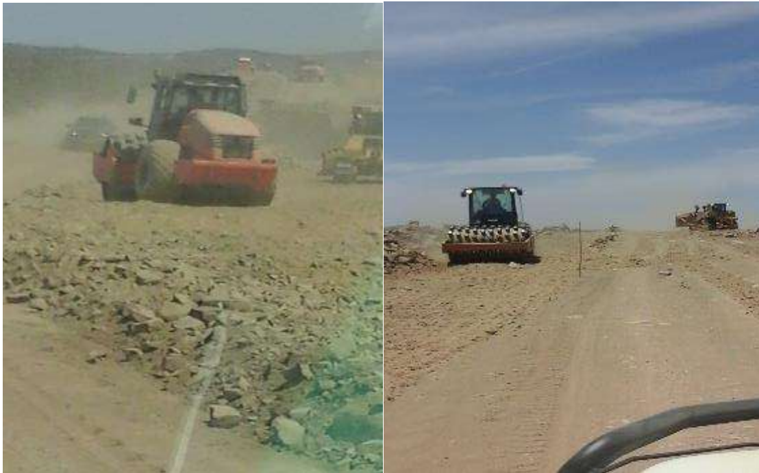
Figure 6: Bulk earthworks in progress (opening access road to facilities)
