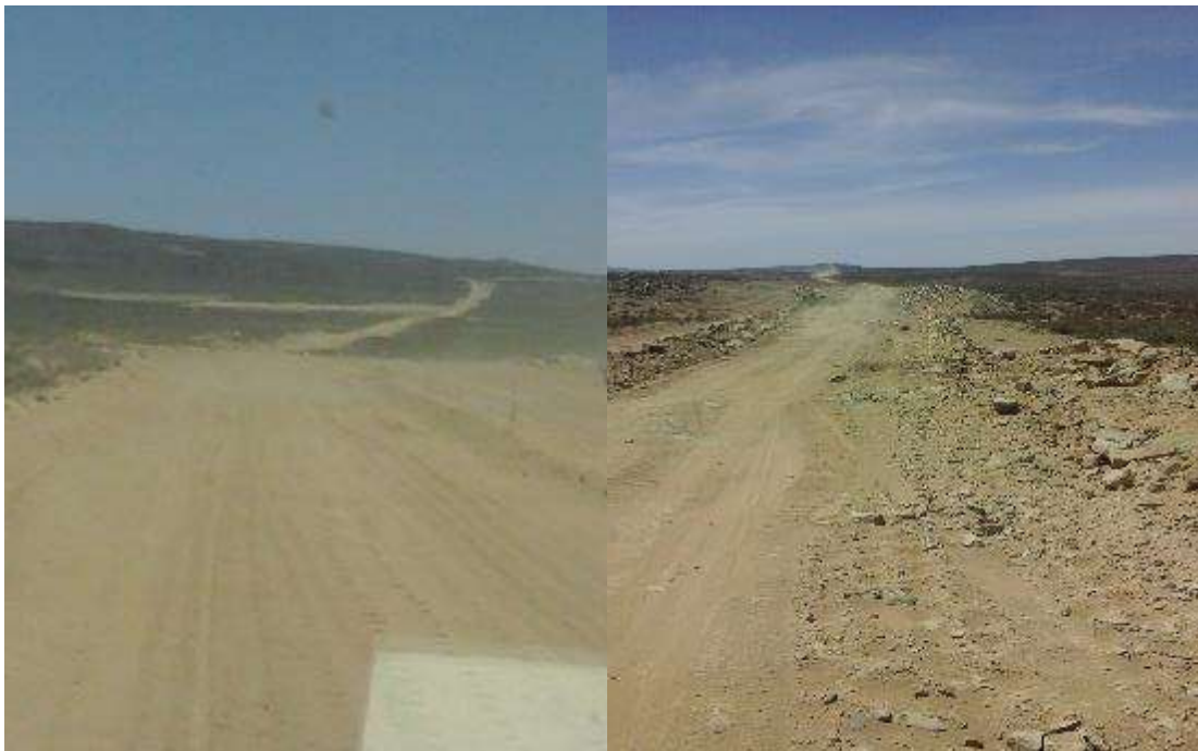
Figure 11: View of recently established access roads.
