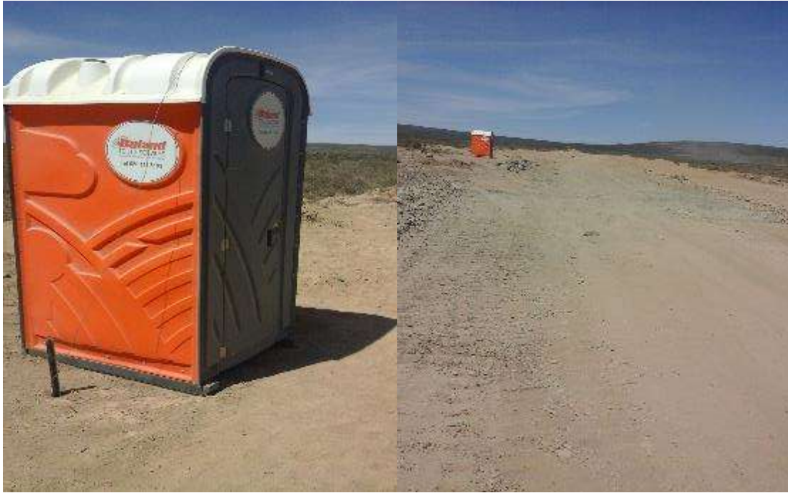
Figure 16: Provision of chemical toilets on site.
