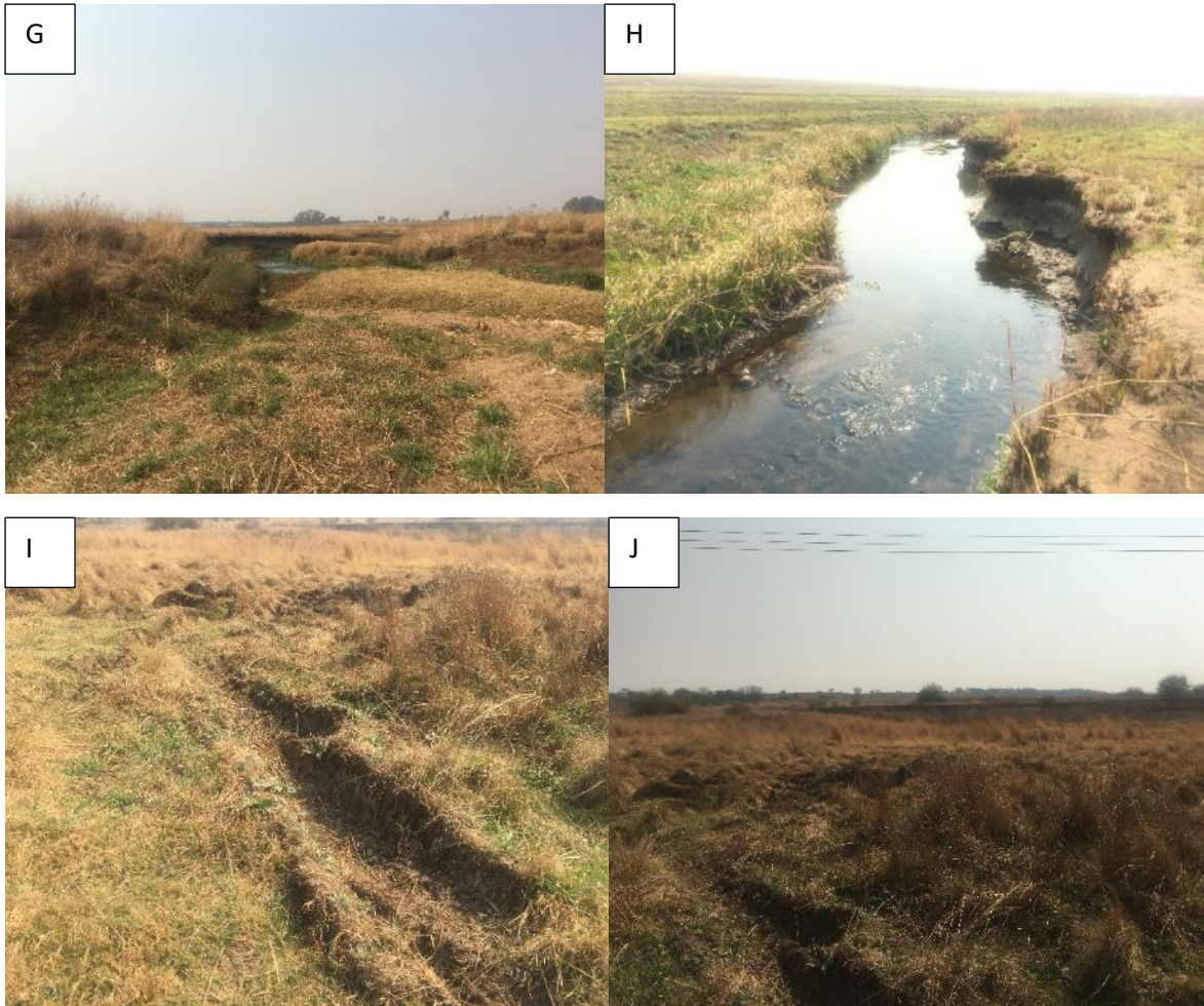
Figure 5: Photographs indicating impacts observed (veld fire, traces of sewerage, water hyacinth, erosion, informal crossings or vehicle driving)
