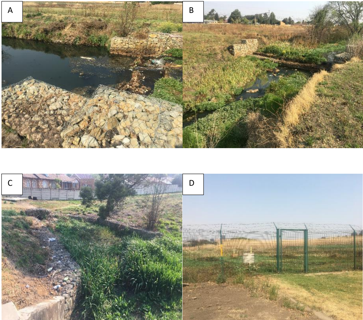
Figure 3: Photographs indicating existing wetland rehabilitation interventions (gabions, fencing off)
