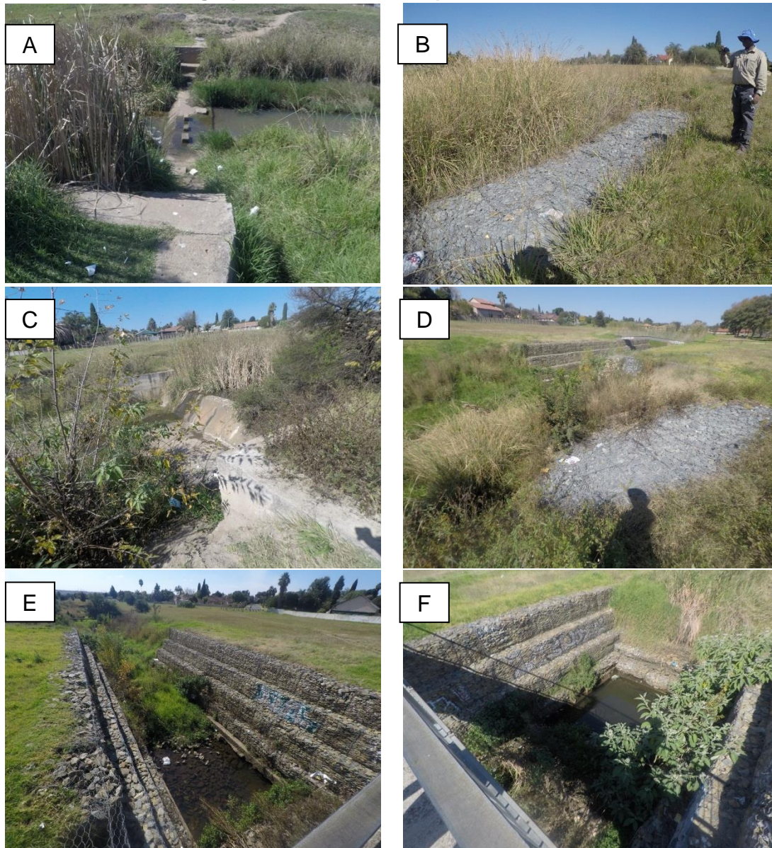
Figure 20: A. Concrete buttress weir (26°2'47.61"S; 28°13'16.44"E); B. Gabion mattress (26°2'48.04"S; 28°13'16.36"E); C. Concrete buttress weir (26°2'54.47"S; 28°13'17.03"E); D. Gabion mattress (26°2'58.56"S; 28°13'17.33"E); E. Gabion weir (26°2'59.46"S; 28°13'17.55"E); F. Gabion weir (26°2'59.46"S; 28°13'17.55"E).
